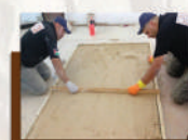
6- Applying Mosaic on the Mortar
