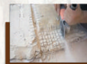
3- Remove Old Cement Support
