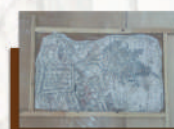
4- Applying Clay as a Temporary Support
